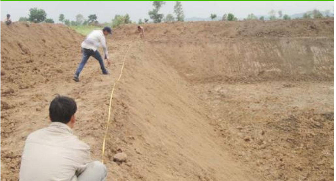
Canal and pond digging activities
